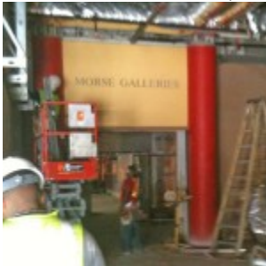
Harbor Hall | August 8, 2011 | Photo: USFSP/John Trecastelli
