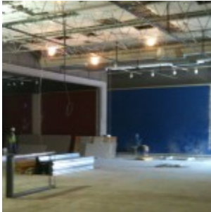
Harbor Hall | August 8, 2011 | Photo: USFSP/John Trecastelli
