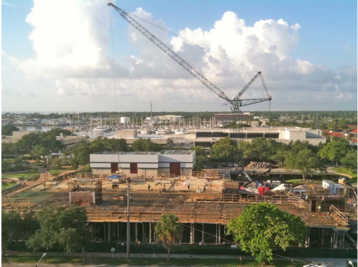
University Student Center 2nd story flooring added
